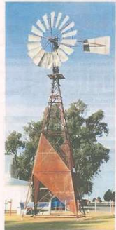
The erection of this windmill was a project of Edward River Council. Constructed by Williams Contracting, Tim and his father, John put up the windmill at Pottinger Park in Conargo. Image credit: Tim Williams Contracting
